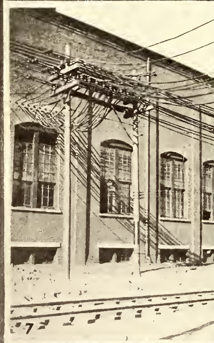
View 1.—General view of Seaview Avenue, showing pole lines which had to be moved back 2 ft. on account of widening of the street.
